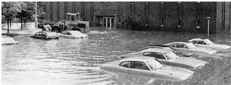
1978 flooding of the ground floor and parking lot of the
